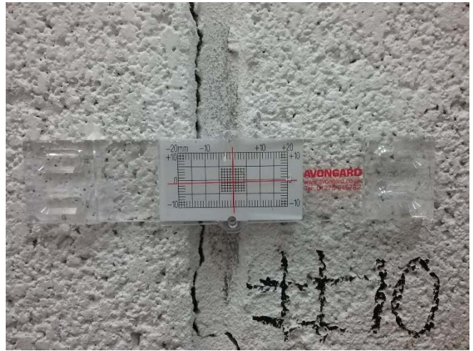
Photo 20: Close up view of crack gauge 10.
