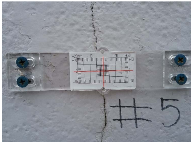
Photo 10: Close up view of crack gauge 5.
