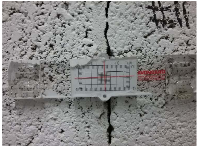
Photo 22: Close up view of crack gauge 11.
