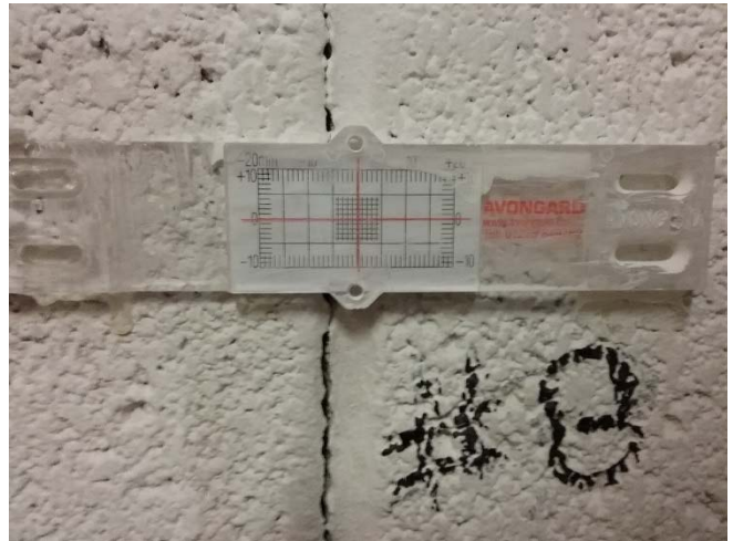
Photo 16: Close up view of crack gauge 8.
