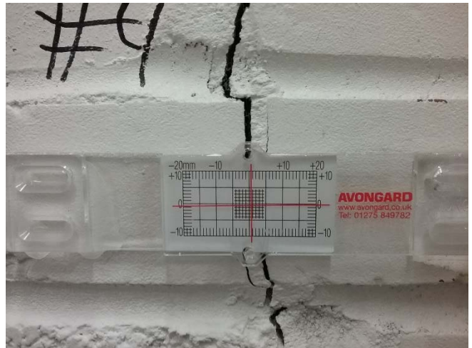
Photo 18: Close up view of crack gauge 9.
