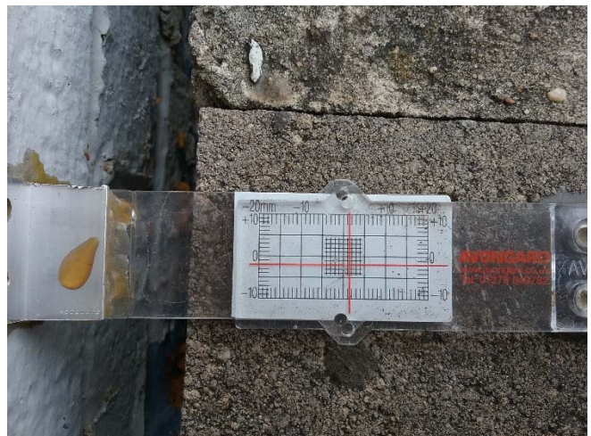
Photo 24: Close up view of crack gauge 12.
