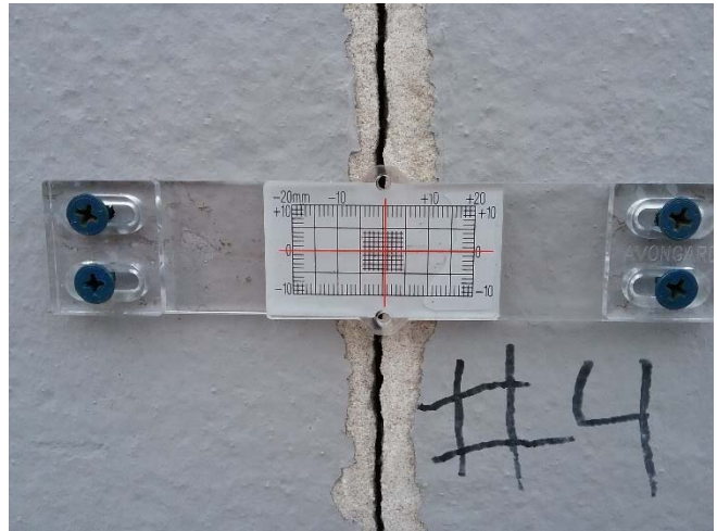
Photo 8: Close up view of crack gauge 4.
