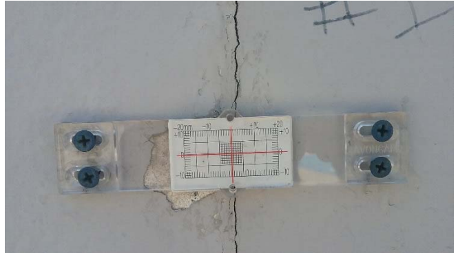
Photo 2: Close up view of crack gauge 1.
