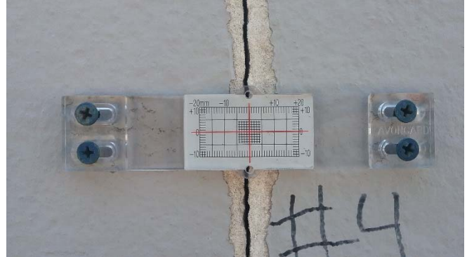
Photo 8: Close up view of crack gauge 4.
