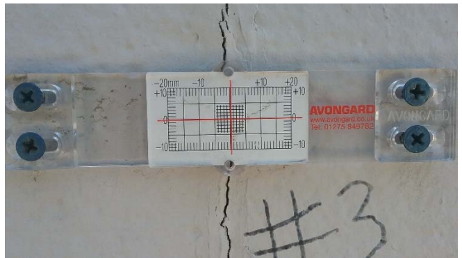
Photo 6: Close up view of crack gauge 3.
