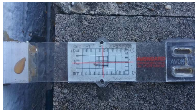
Photo 24: Close up view of crack gauge 12.
