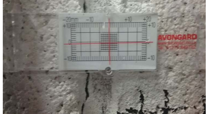
Photo 20: Close up view of crack gauge 10.
