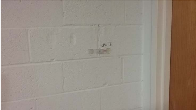
Photo 13: Crack gauge 7 position in an interior storage room.
