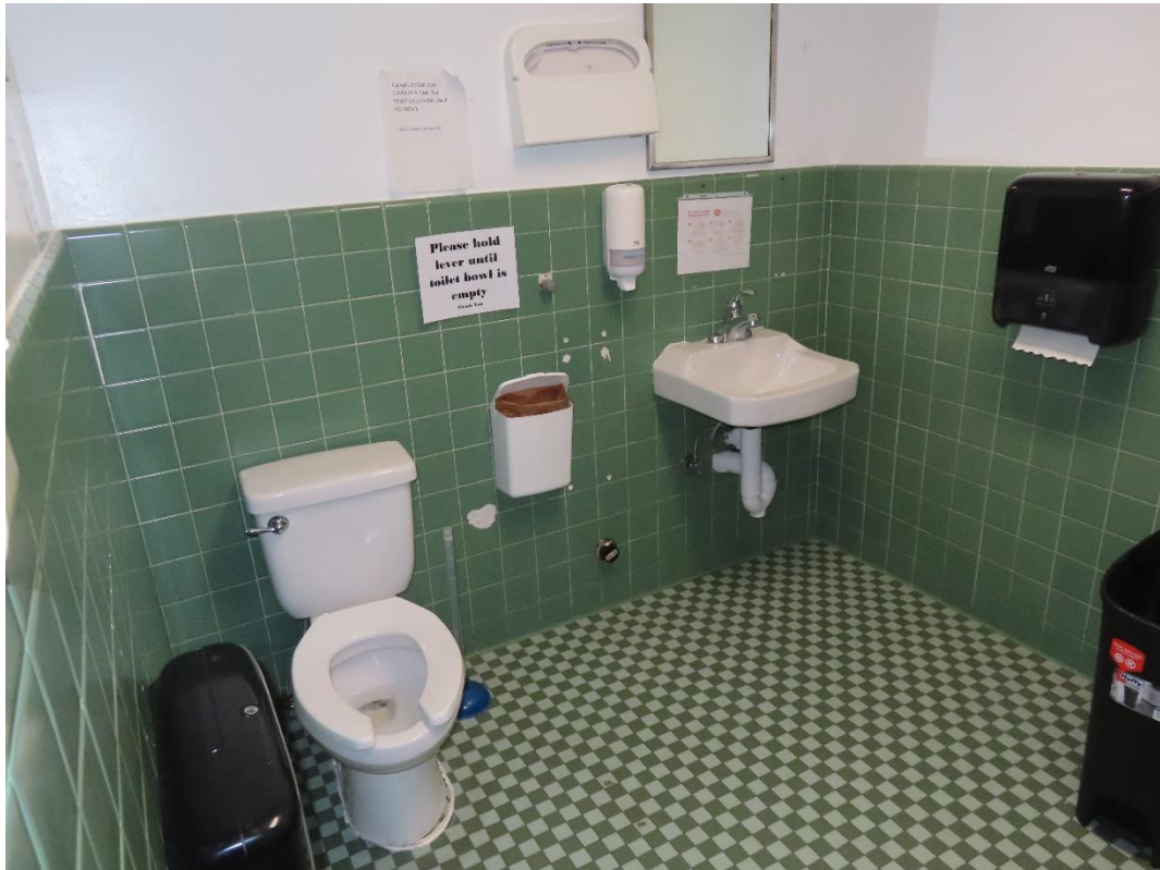
Photograph 3: Add grab rails to make ground floor accessible rest room fully accessible.
