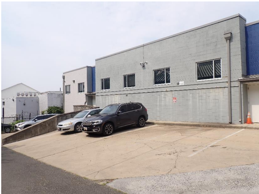
Photograph 22: Exterior wall systems and finishes.
