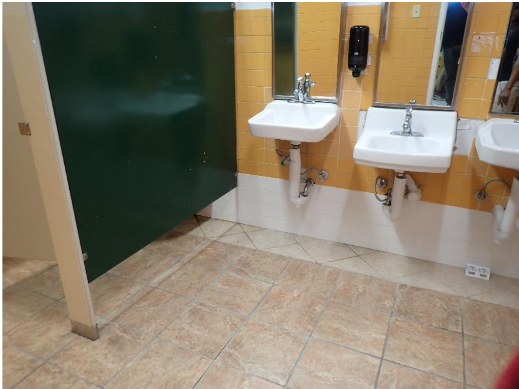
Photograph 26: Typical bathroom finishes.
