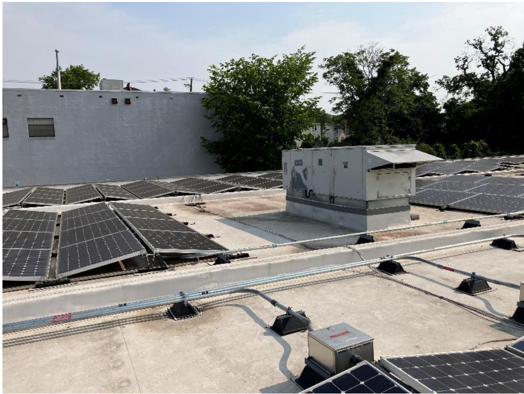
Photograph 16: Overview of roof.
