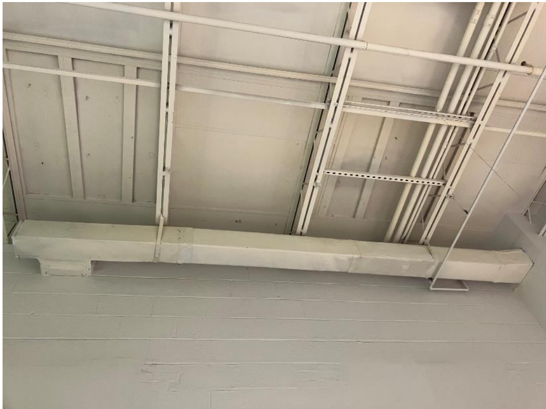
Photograph 12: Roof structure viewed from inside.
