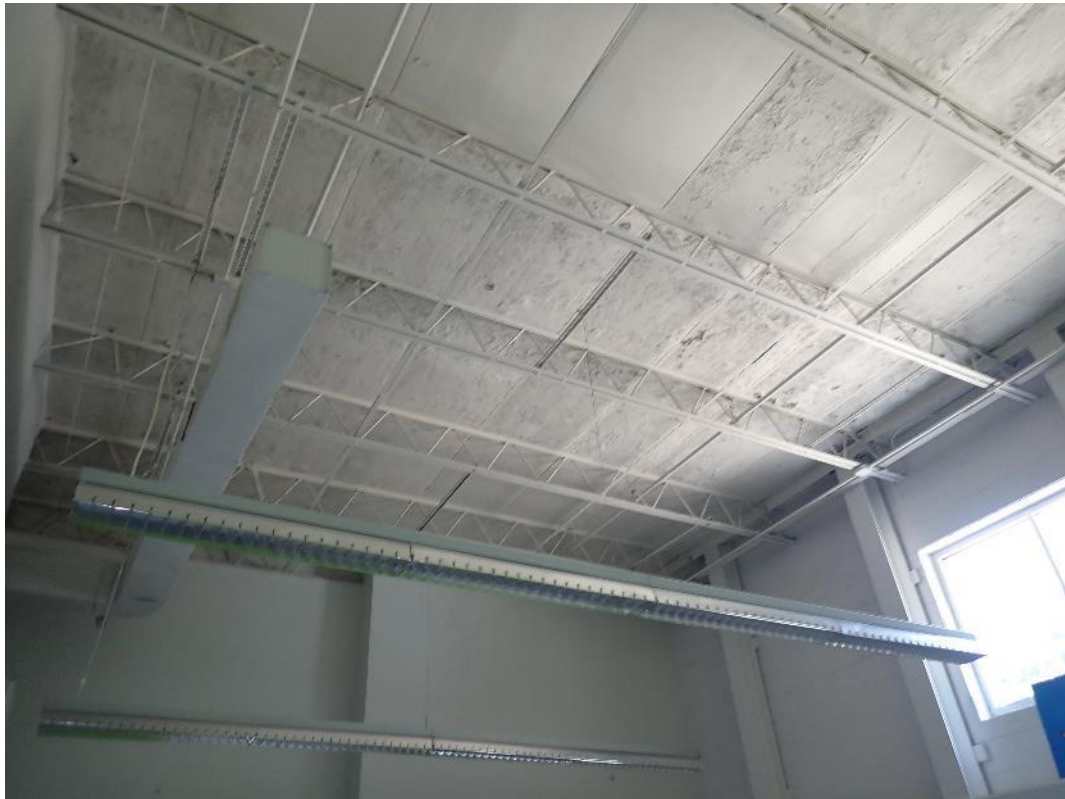
Photograph 13: Roof structure viewed from inside at classroom area
