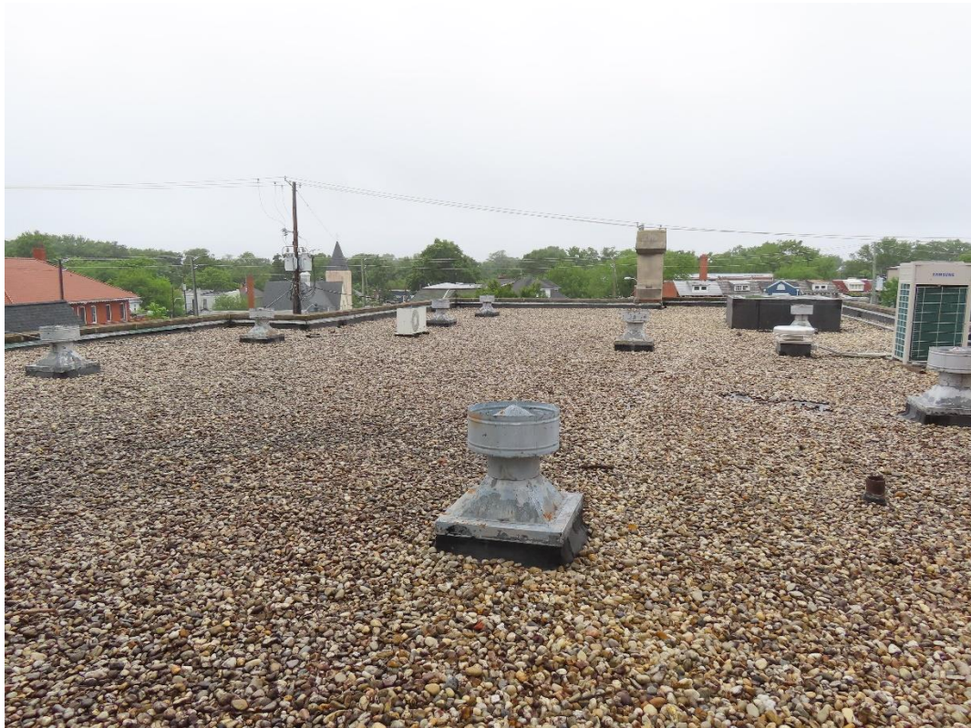
Photograph 10: Ballasted EPDM roof.
