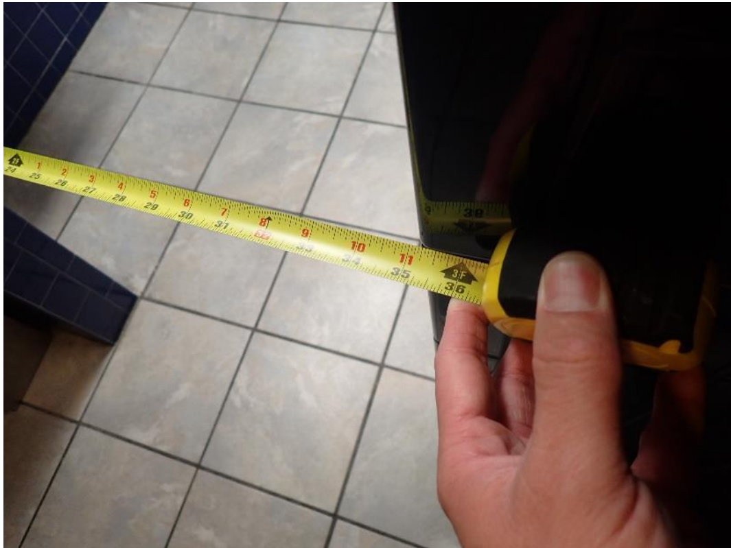
Photograph 5: Compliant clear opening at restroom door.
