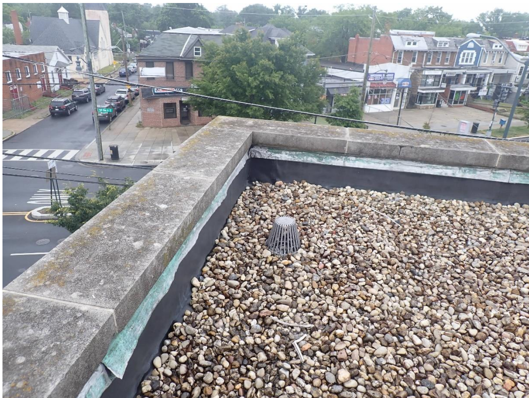
Photograph 20: Stone parapet and copper flashing.
