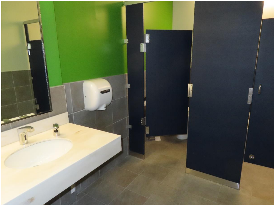
Photograph 46: Upgraded ADA restroom.
