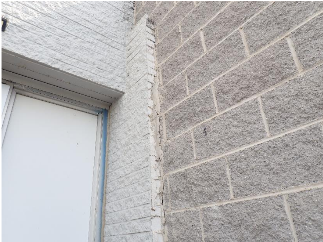
Photograph 21: Brick and split-face CMU walls.
