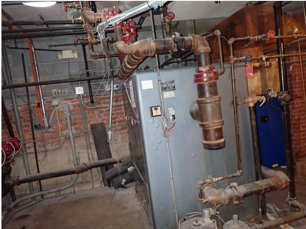
Photograph 25: Hydronic boiler.
