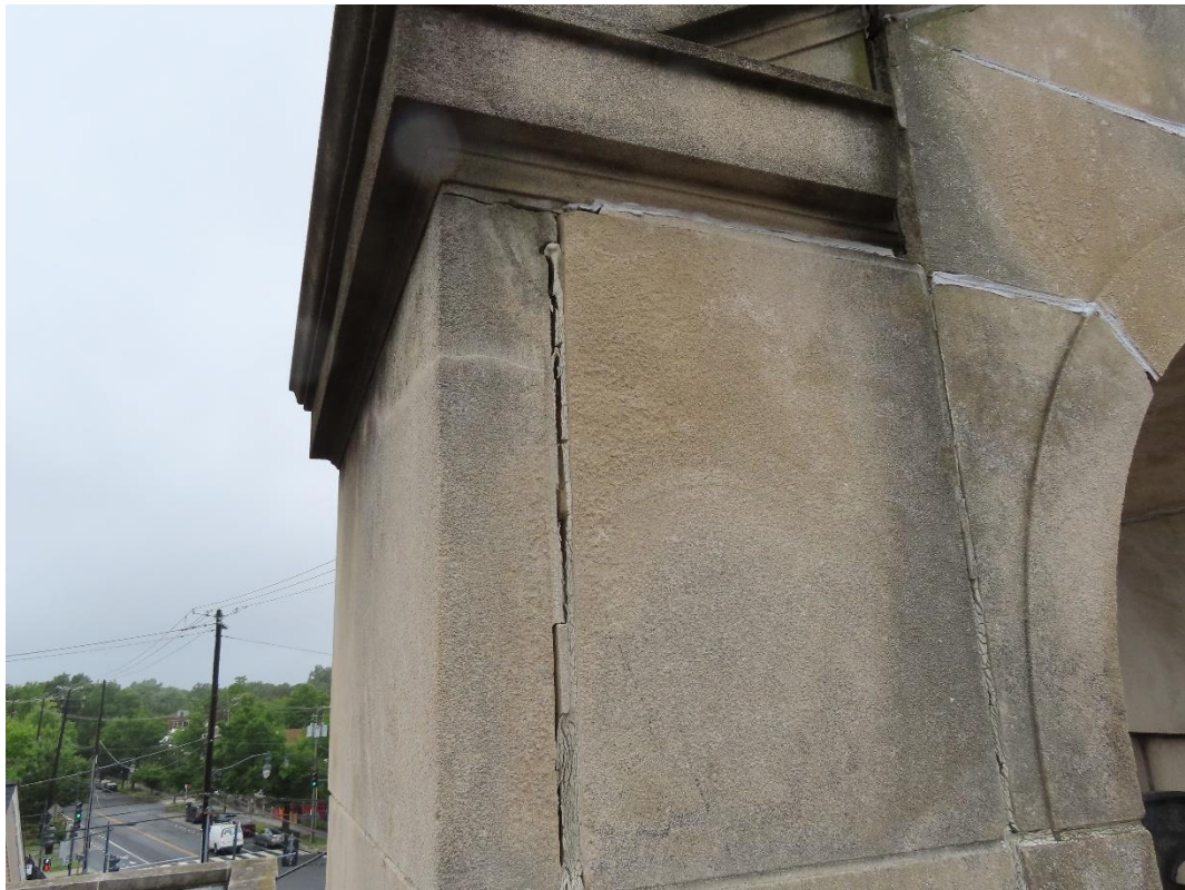
Photograph 16: Movement of stone panels to bell tower.
