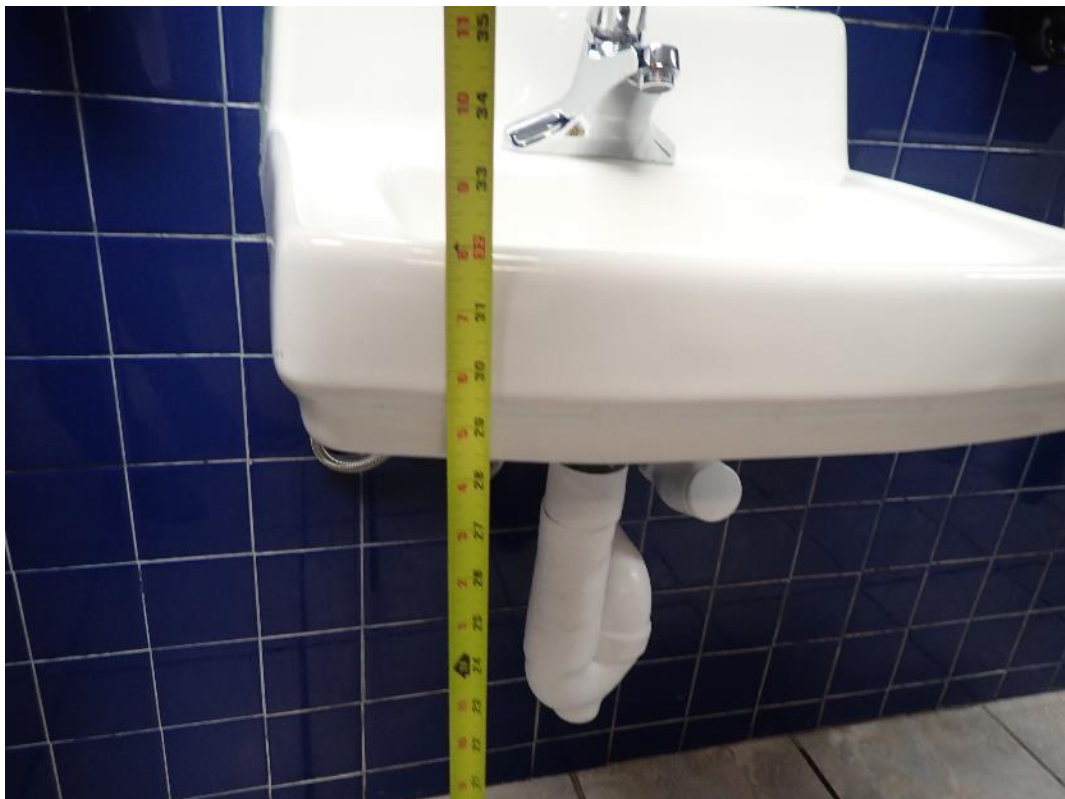
Photograph 4: Compliant lavatory in restroom.
