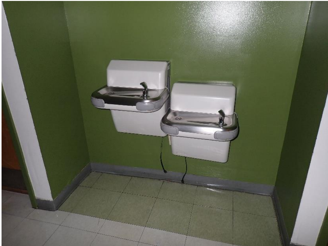
Photograph 1: Split level water fountain.
