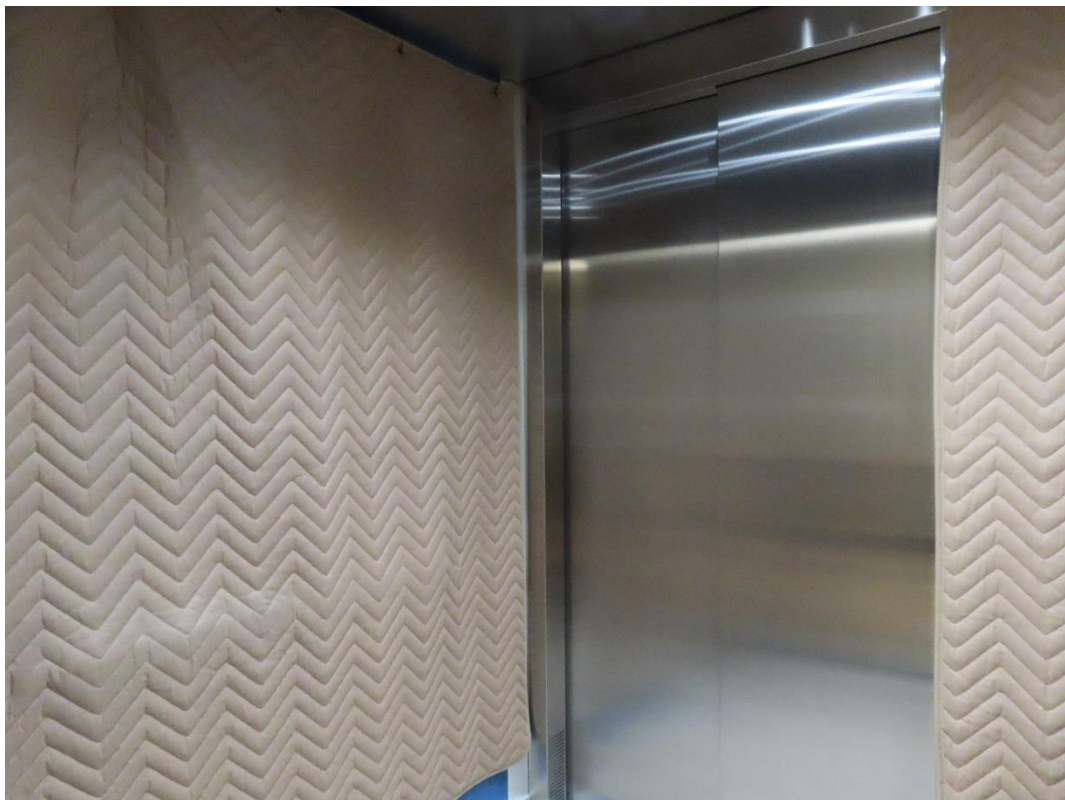
Photograph 54: Elevator cab interior.
