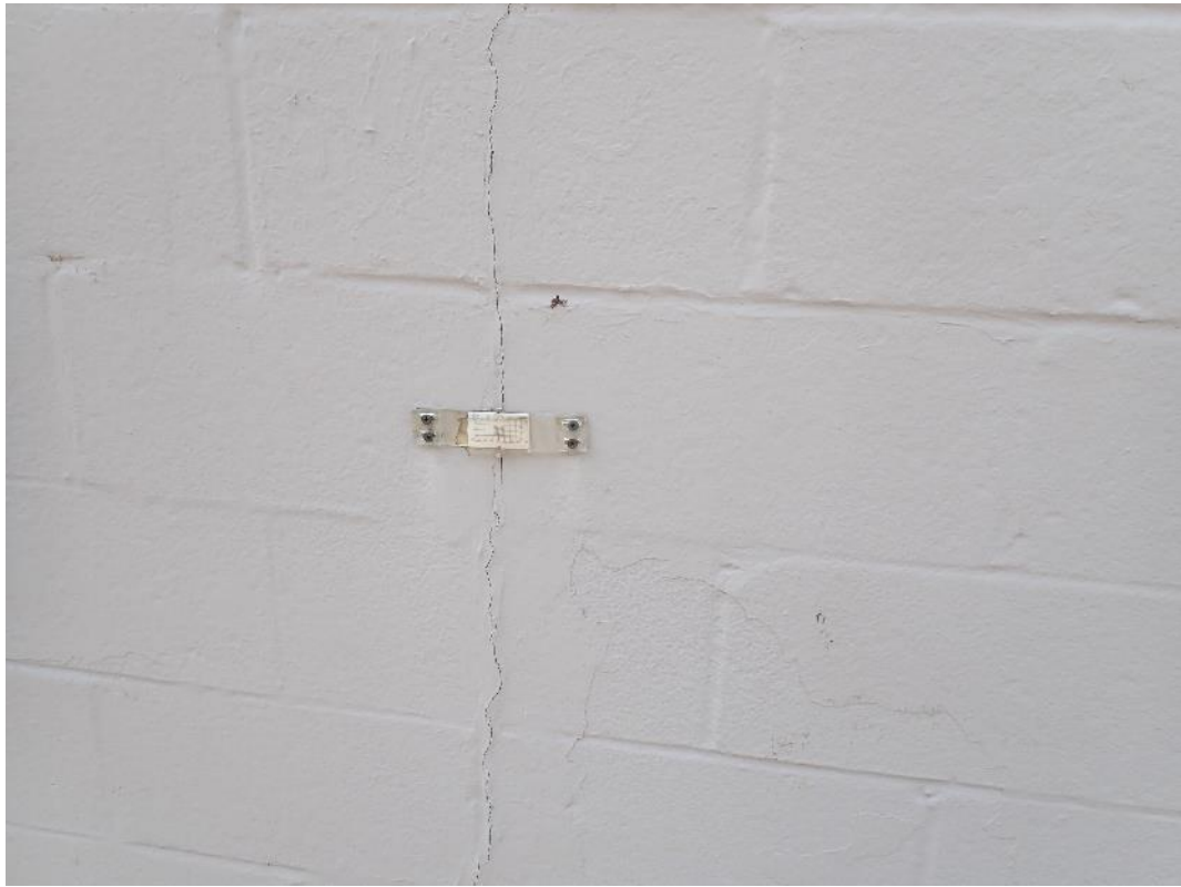
Photograph 15: Crack gauges on exterior wall from previous crack monitoring.
